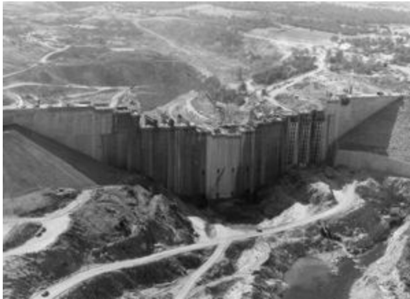
Folsom Dam Construction, 1955
