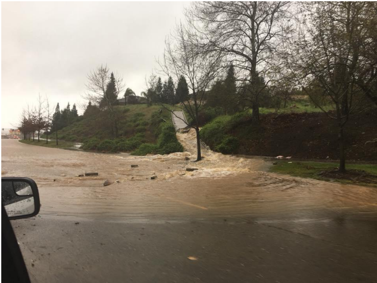
Figure C-24 2018 Flooding – Iron Point East of Cavitt
