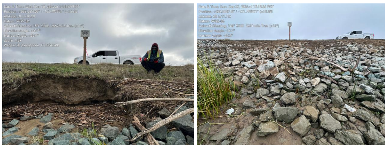
Figure 4-3 December 2024 – Emergency Repairs on Levee Before and After
