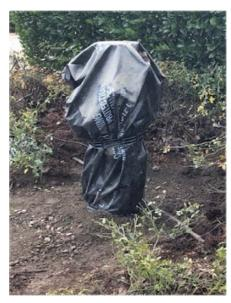
Fire hydrants that are not in service yet, shall be covered with a **black plastic bag**. Once the hydrants are in service the plastic bag will be removed.
