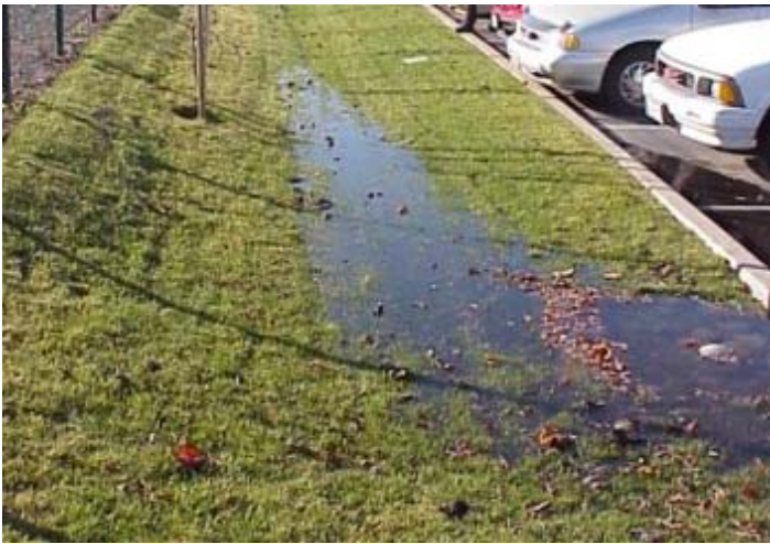
Cal Expo Swale. Learn about the benefit of using vegetated swales with a convenient online video.
