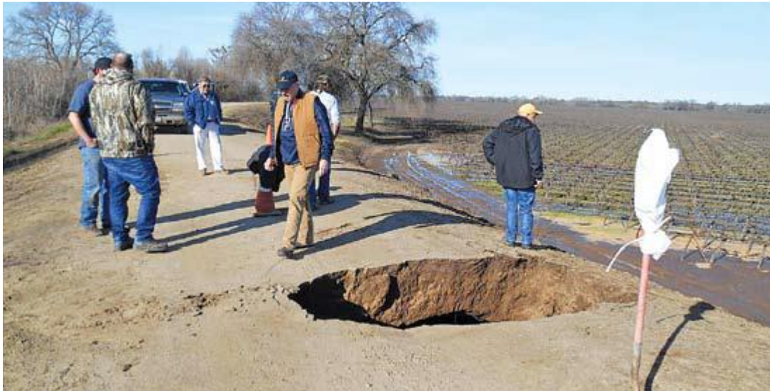
Figure K-3 RD 800 – Levee Boil
