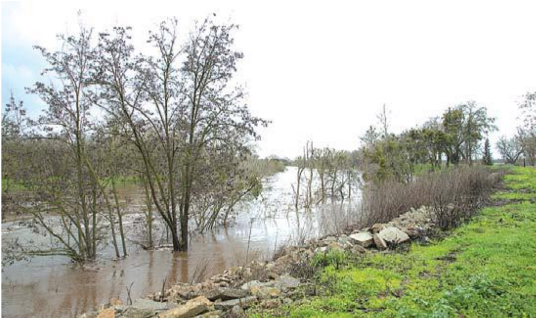
Figure K-4 RD 800 – High Water from 2017 Storms
